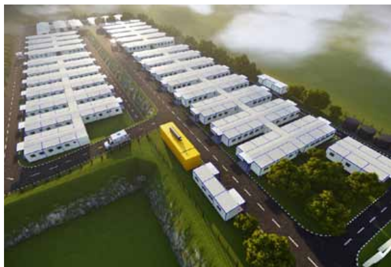
Tata Projects is constructing a medical facility at Kasaragod in Kerala with 80-quarantine rooms comprising 551 beds as part of its plan to augment hospital infrastructure across India
